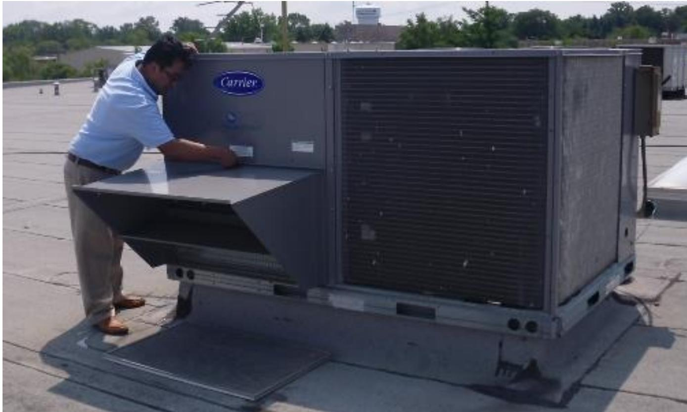
*Contemporary Controls outfitted four dual-stage heating/cooling RTUs with economizers on the roof of the company's Downers Grove, IL facility with CvRTUv2 programs. All units are scheduled using a variety of head-ends for testing purposes.*
