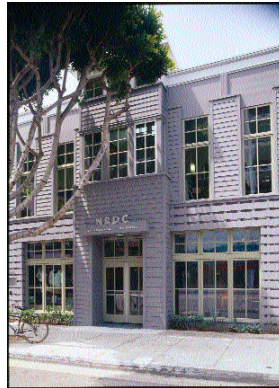
This photo shows the entrance to the NRDC's new office in the Robert Redford Building. Facility renovation spanned eight months. (Photo courtesy of Tim Street-Porter and the NRDC)
